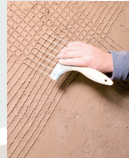
Scratch coat being scratched with a wire comb/lath scratcher!
