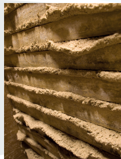
Nibs forming at the back of the laths give a 'finger hold'
