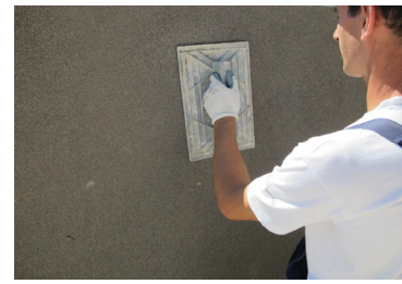
Trowelling of final surface
