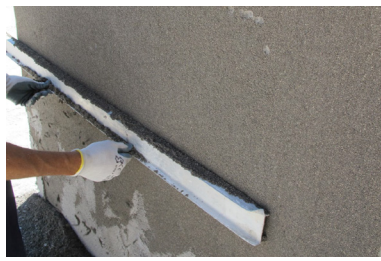
Levelling of surface with ruler
