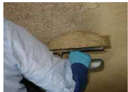
Applying lime hemp plaster (base coat) to wood wool boards.
