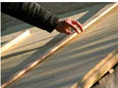
Installing sarking board over rafters.
