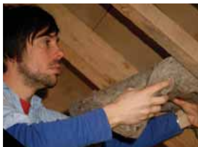
Placing sheep's wool insulation between rafters and under sarking board.
