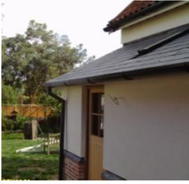
*Lime plasters need damping down to control the carbonation of the lime however, Fibrelime does not have the same degree of reliance on this, but it is good practice to moisture control it under dry conditions in order to get the best from the product.*
