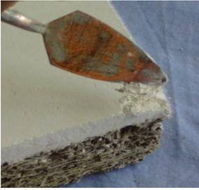
*Fibrelime finished plaster requires minimal maintenance, simply damp the plaster and fill any impact damage or movement cracks, with more Fibrelime, clean down all powdery residues and repaint.*
