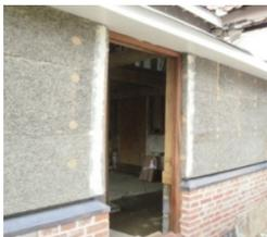
***It is essential that Fibrelime is mixed very well***, preferably using a paddle mixer, this will ensure that the ingredients are properly re-blended and that the plaster is suitably 'fat' which results in a more workable material. Failure to carry out remixing will affect the performance and ease of application.
