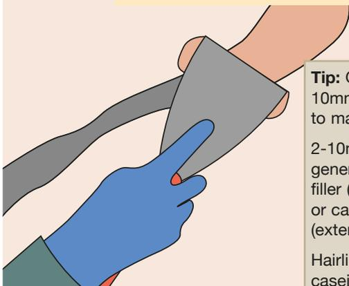
**Tip:** Greater than 10mm = lime plaster to match existing
