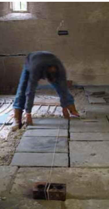
glaster® screed was chosen by the National Museum and Galleries of Wales for their under floor heating carrier before laying the flagstones on their insulated limecrete floor in the 13th Century Church at St Fagan's.
