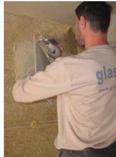
Internal glaster® plaster being applied to Ty-Mawr wood wool boards.
