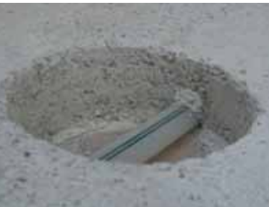
A heating pipe in the glaster® screed
