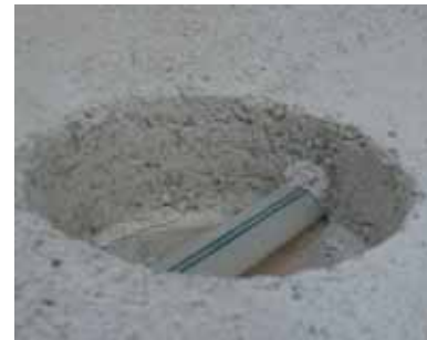
A heating pipe in the Glasscrete Screed.
